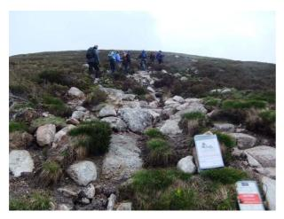
Cairngorm Wilderness Contracts have been awarded the contract for the Sron na Lairig section. This includes work on deep, steep peat on the lower part where a full-build solution of block pitching and aggregate is being used, through to lower impact (light touch) work to define a preferred line on the upper section. At the time of the visit the team were completing a stone pitching and undertaking landscaping work. This team is using the Remote Accommodation System.
