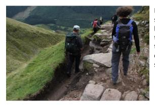
Immediately beyond this, the path degenerated into an appalling scene where only the heavy built pitched path surface and the heavily-built side drains and cross drains had survived. Any path that had been completed as aggregate had washed away, leaving the stonework proud by 30 to 60 cm. In two places, turf had been eroded to depths estimated to be around one metre. A substantial section has been let as a contract which will begin in October.
