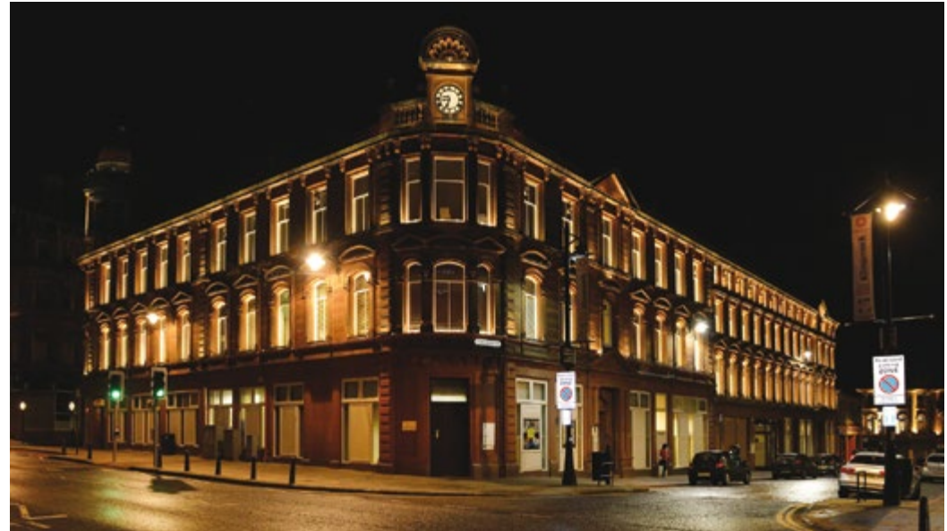
Civic Centre, John Dickie Street, Kilmarnock
