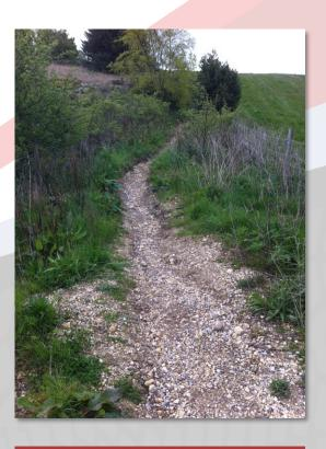
Above: The naturally formed path was also a nuisance for pedestrian users and cyclists, having gone past the point of being rugged terrain and in to the realms of being unsafe. Below: The steep incline and rainwater run off had combined to erode the bridleway, making it unsafe for riders to take horse on to the Folly Lane stretch. Note the collapsed drainage pipe (circled) that was previously installed in an attempt to alleviate the erosion.
