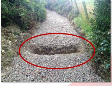
This page: Having widened the existing path, baffles were dug in to the steeper inclines to allow water to effectively recharge back into the ground after penetrating through the KBI Flexi<sup>TM</sup>-Pave. The baffles (circled) also reduce the migration of the stone used within the sub-base, helping to ensure a stable path.
