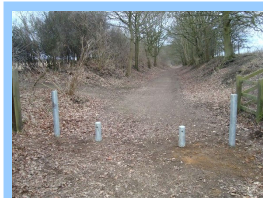
Photo 10 – Kent carriage gap
