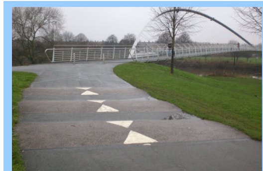
Photo 7 – Speed humps on cycle track (York)
