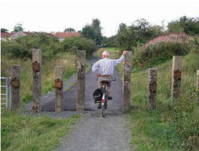
Sleepers used as bollards on NCN 73, Ayrshire
