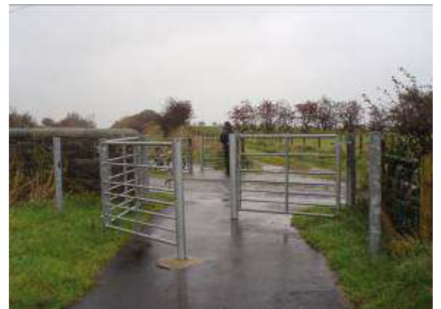
Removable central gate post to allow maintenance vehicle access on NCN 7
