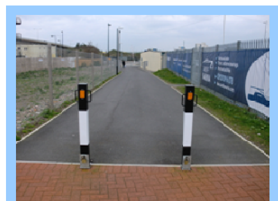
Photo 4 – De-mountable bollards to enable maintenance access (Cardiff)
