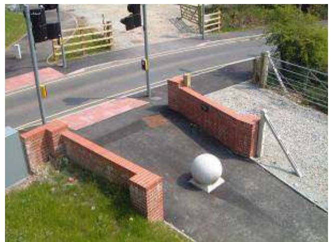
Central bollard with ample passing space and adjacent maintenance vehicle access gate
