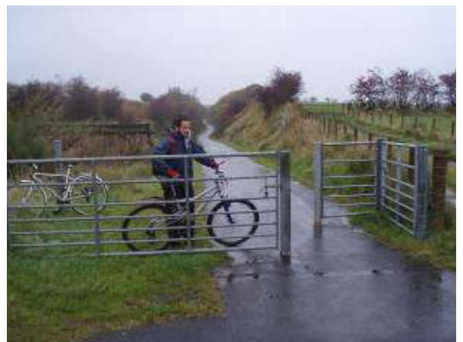
Locked maintenance vehicle access gate incorporated into chicane on NCN 7
