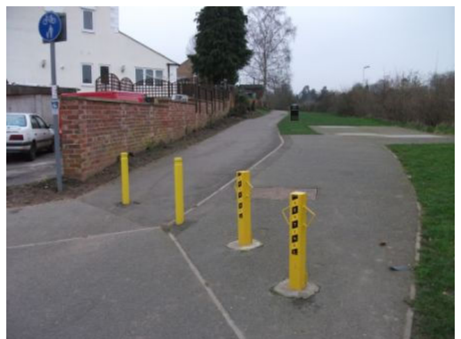
Fixed and demountable bollards
