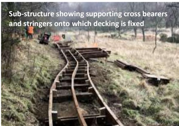
Decking boards were spaced at 5mm and toe boards were installed along each side; for wheelchair users or people with mobility difficulties who may feel less comfortable being on a raised boardwalk.
