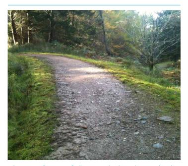
The surface of the trails had eroded in places, and the gradients were too steep for current easy access standards.
