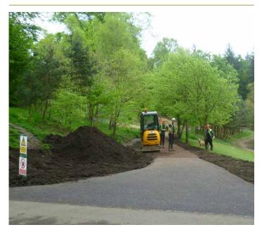
Transition zones between the new path and existing tracks through the wood needed particular attention to maintain the right gradient.
