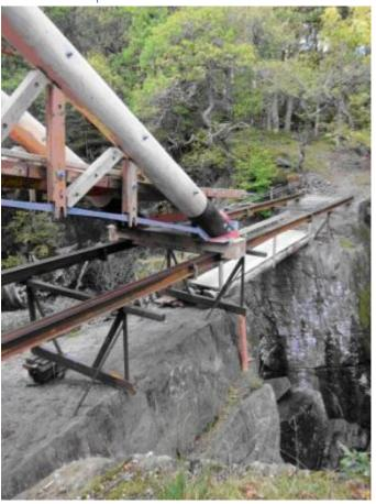
20metre span bespoke steel timber bridge supported by four 12metre Douglas Fir trunks in an A-frame shape with copper roof. Other materials were steel and larch. Ground works included the creation of a new eastern abutment and the carving of a western abutment out of the pudding rock. Installation involved hand winching of completed structure across temporary beams as show in photograph.
