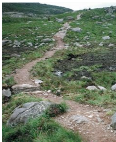
Repaired section of damaged stalkers path; on-site boulders, turf and aggregate used to mimic the original 19th century design. Coire Dubh, Glen Torridon. See path assessment for the path pre-repair work.
