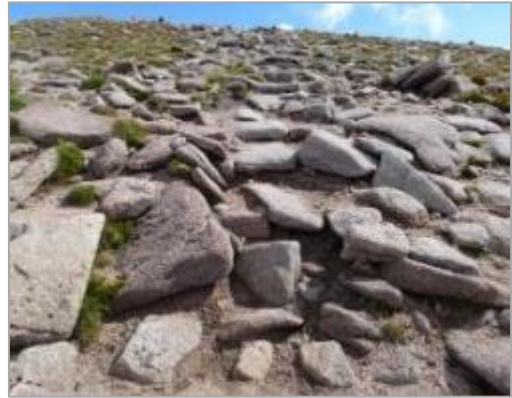
Short flight of pitching designed to look like a natural pile of boulders on Cairngorm
