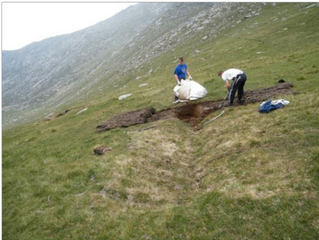
Construction of a turf lined ditch in Coire Lan, Arran
