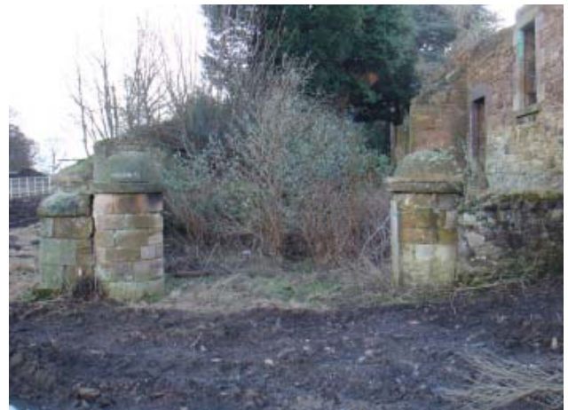
A ruined stable block remains on the site
