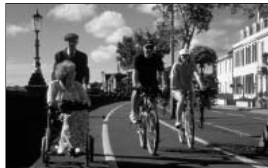
A previously pedestrian-only facility has been converted to shared use, with a raised tactile delineator strip demarcating the pedestrians' and cyclists' sides. Barnstaple, Tarka Trail.
