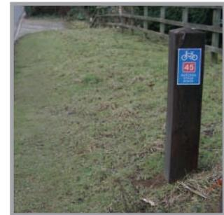
Figure 22: Confirmation sign fixed to a timber bollard, National Route 45
