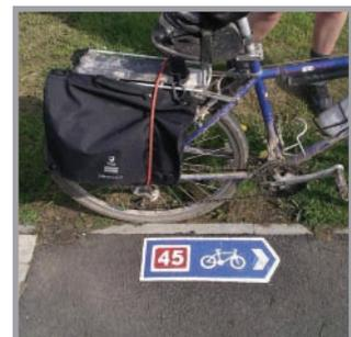
Figure 24: Preformed thermoplastic marking on traffic-free section of National Route 45, manufactured by Preformed Markings SW
